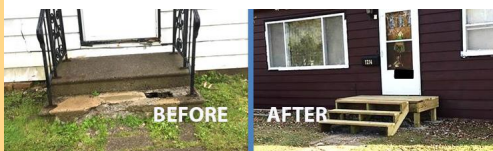
HIP improvements create a safer entryway
